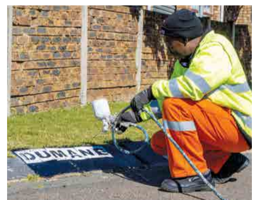
Municipal employee repainting street names.
