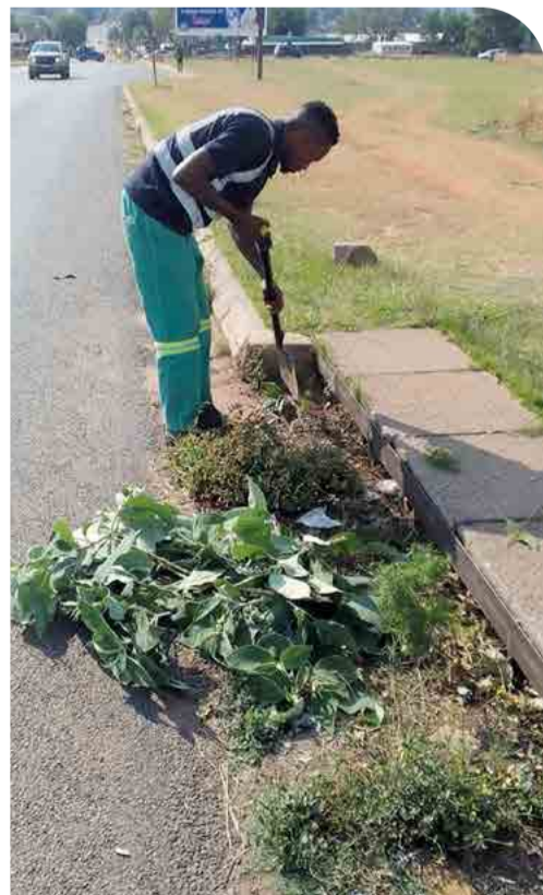
Removing weeds blocking stormwater drains.
