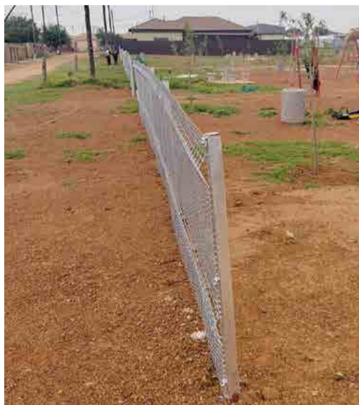
Clear view fence.
