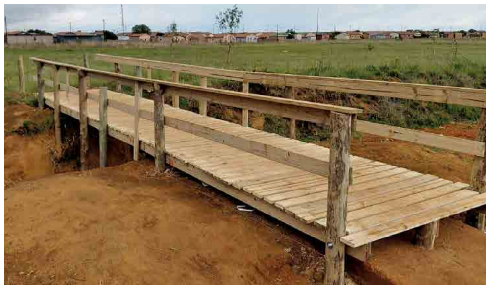
Wooden foot bridge to access the park in Rockdale Ext 2.
